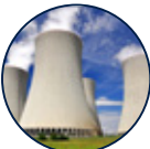
Cooling Tower Water
